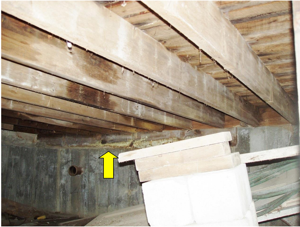
Facing east from bulkhead. Yellow arrow points to damaged section of sill.
