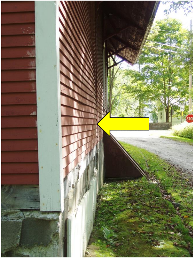
Facing south toward west elevation, yellow arrow points to bulge in wall
