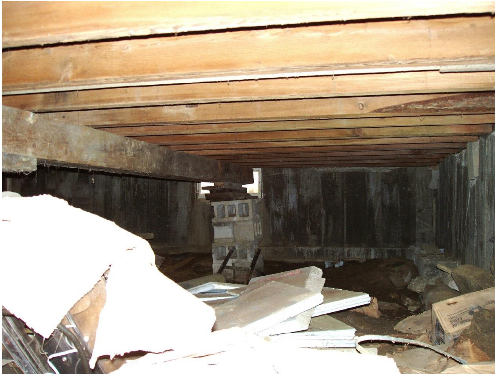
Facing south from bulkhead. Note insufficient beam support.
