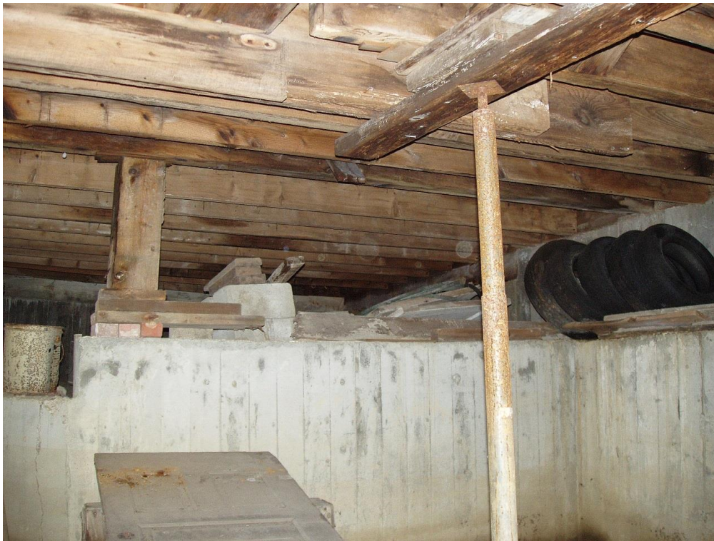
Facing northeast from bulkhead. Note insufficient beam support.
