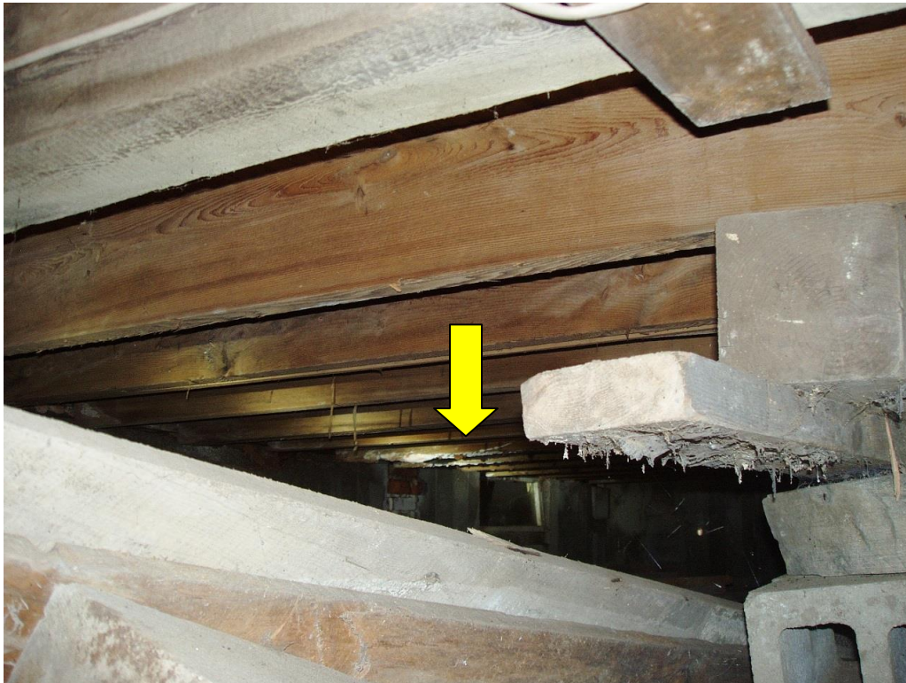
Facing southeast from bulkhead. Yellow arrow points to damaged sections of joists.
